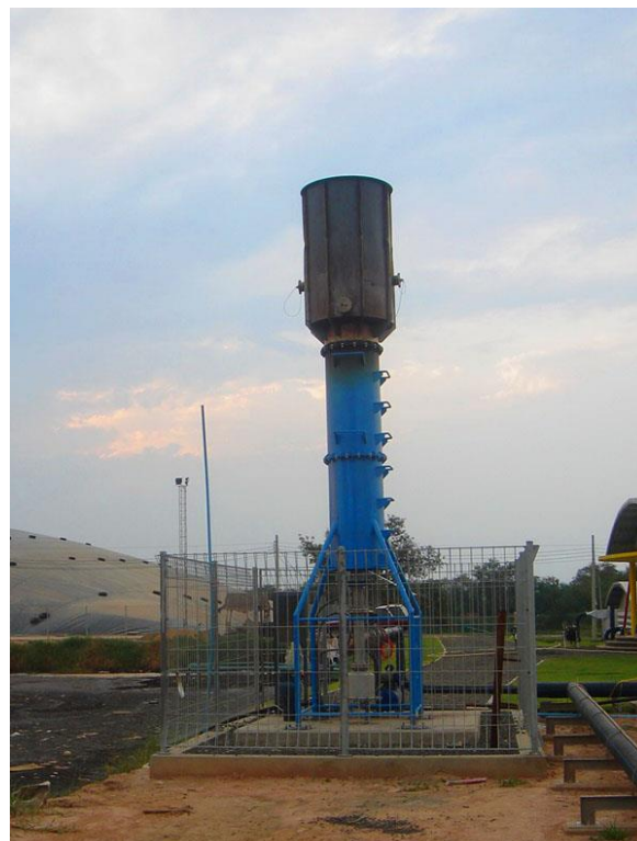
Figure 1.2: The proposed initial start-up blower and a 1000 Nm3/h flare station.
